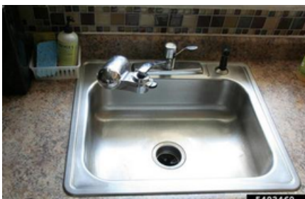
Drains without screens
